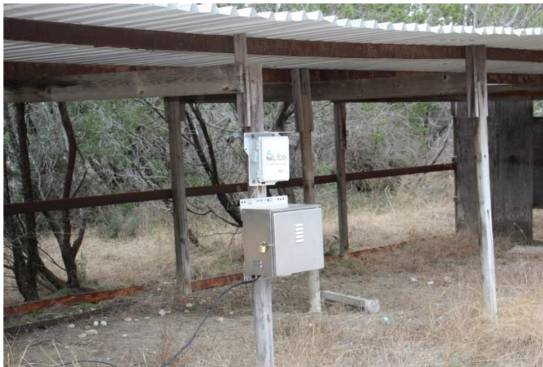
Exhibit 5 Installation of Monitor at Southern Site
