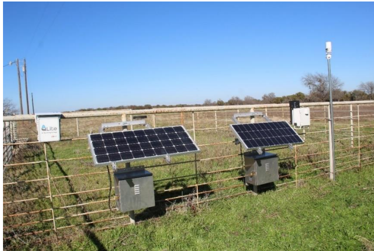
Exhibit 2 Installation of Monitors at Northern Site
